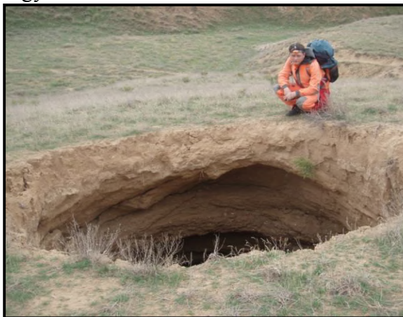
Figure 1 - Suffosion and karst failure in Sharovskaya gully (photo by I.V. Golovachev)
