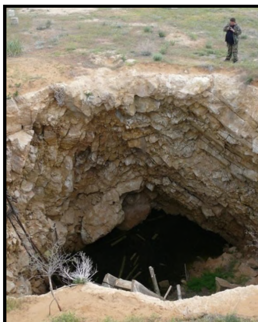
Figure 21 - Faulty well (Photo by A.A. Shaposhnikov)
