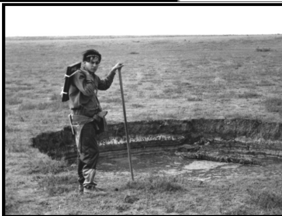
Figure 8 - Failure at Gorky Lake in 1994. (Photo by I.V. Golovachev)
